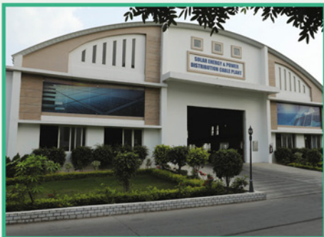
Solar Energy & Power Distribution Cable Plant at Rewa (M.P.)
