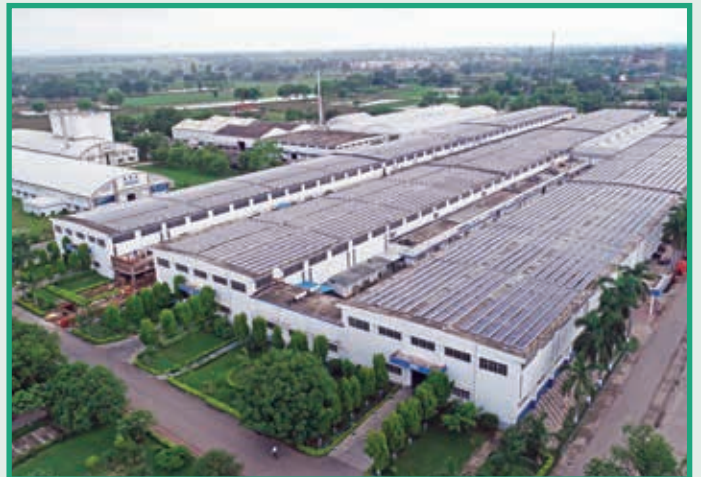
VTL Plant - Aerial View at Rewa (M.P.)
