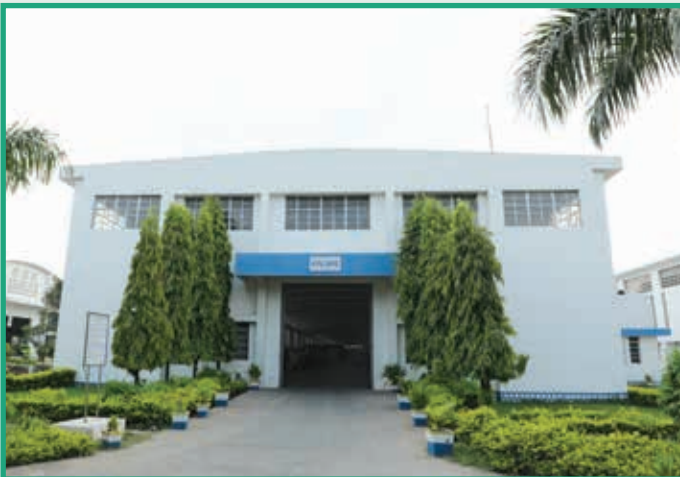
VTL - OFC Plant at Rewa (M.P.)
